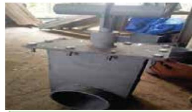
**AFBC Boiler Bed Drain slide gates.**
